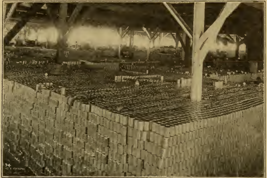
FIG. 43. — Interior of a salmon cannery.
